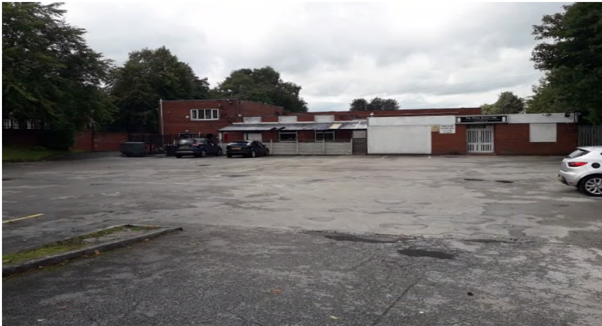
Existing Whitehouse club building with car parking to the front fronting on Middleton Road
